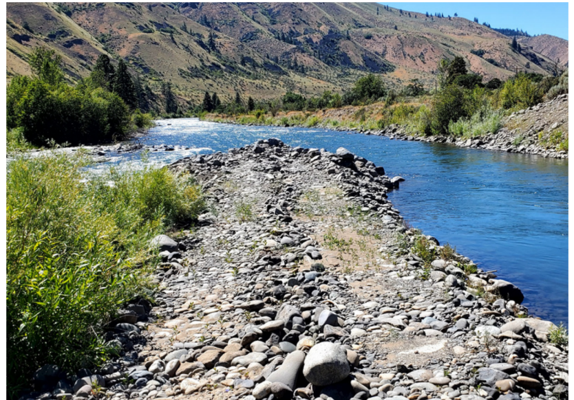
View of the Naches River diversion looking west, upstream.
