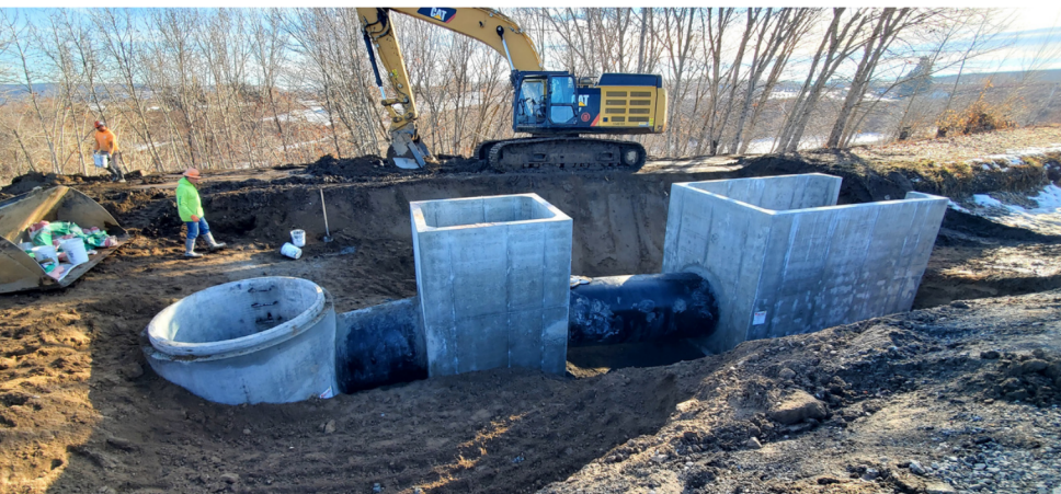
Precast concrete structures leading from No. 3 Lateral canal
